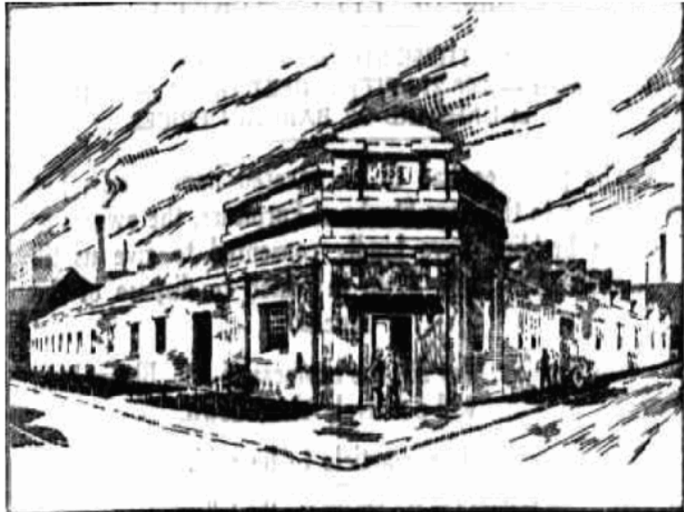
COMMONWEALTH WEAVING MILLS FACTORY AT WATERLOO.
